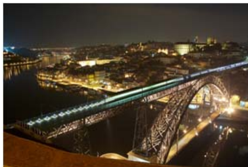
Douro River and D. Luís metallic bridge engineered by Théophile Seyrig a Gustave Eiffel disciple
